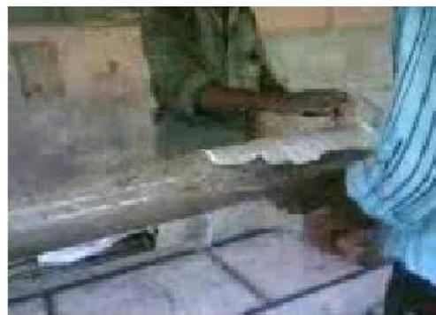
**Fig. 2. GFRP Wrapping under Progress**
